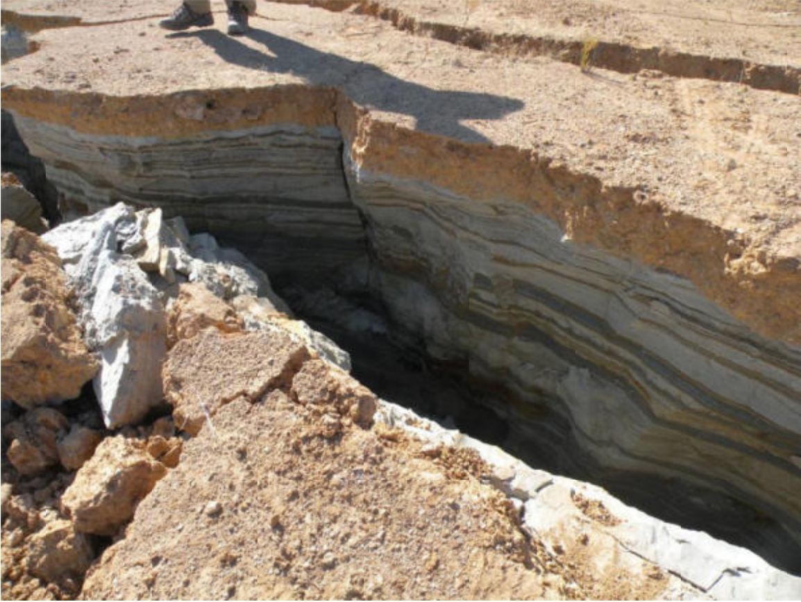
Figure 3.5 Gravelly cover layer over oxidized and unsaturated tailings, S35.184679 S, W71.759410 (from GEER [2010]).
