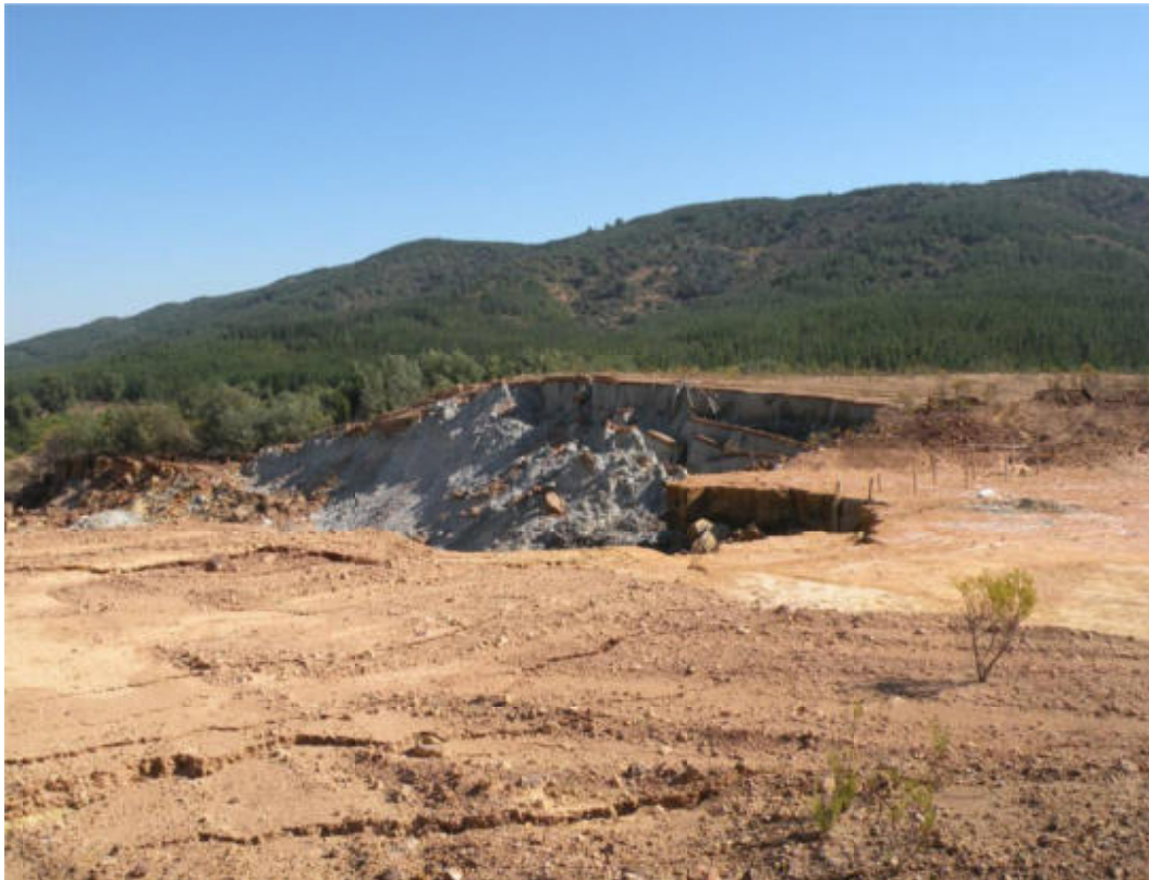
Figure 3.1 Upper scarp of failed tailings impoundment looking southwest (from GEER [2010]).
