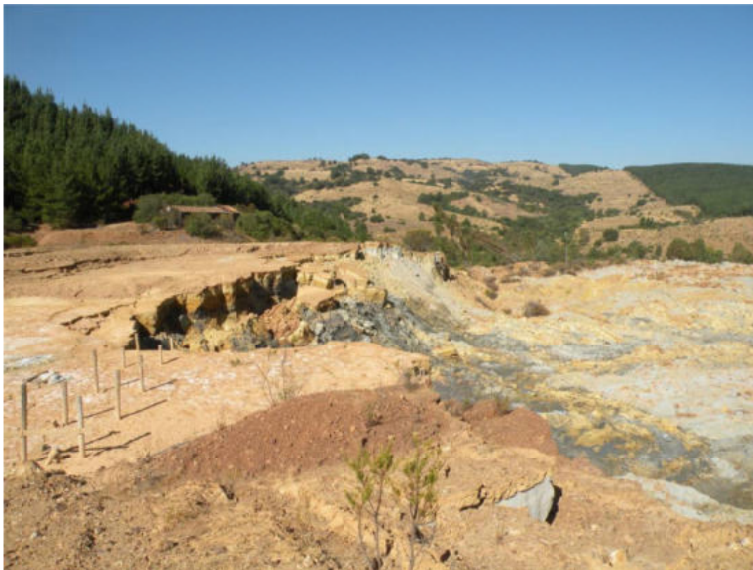
Figure 3.2 Upper scarp of failed tailings impoundment looking northeast (from GEER [2010]).
