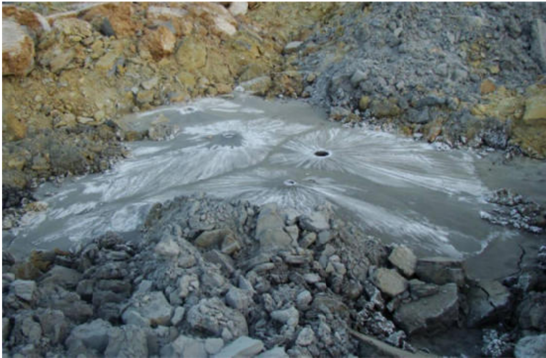
Figure 6.2 Evidence of sand boils in the flow-failure debris (from GEER [2010]).
