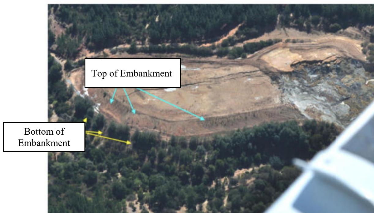
Figure 3.3 Aerial photograph showing scarp, longitudinal cracks, and the location of the tailings dams (after DICTUC [2012] and Gebhart [2016]).
