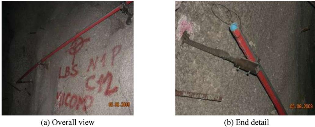
Fig. 6 Sensor tubes attached to the tunnel sidewall
